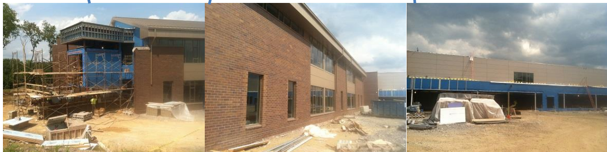
Figure 3: Construction Progress Photos (Property of Mascaro Construction)
