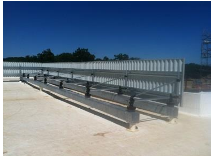
Figure 7: TPO Roofing & Roofscreen Photograph taken from Area B Roof (Property of Mascaro Construction)
