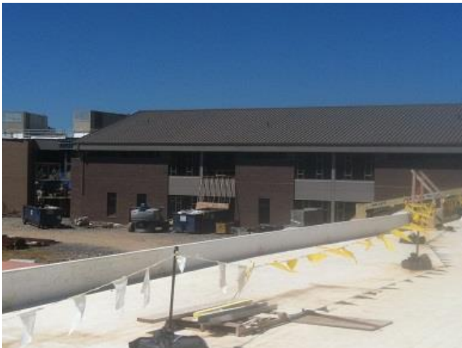
Figure 6: Standing Seam Metal Roofing Photograph from Main Corridor Roof on Area F (Property of Mascaro Construction)
